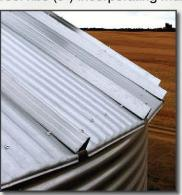
added strength to the roof panels. Sukup even went the extra step of making the ribs two different widths for a better overlap and fit. The inner or lower rib is slightly smaller than the upper, allowing the sheets to nest properly.
