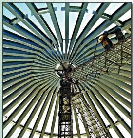
Sukup offers commercial roofs with 15.000, 30.000 or 50,000 lb. peak load ratings. Roof ratings are pounds evenly distributed on peak ring as pure vertical load with uniformly distrubted roof snow load calculated from 40 psf ground snow zone or 90 mph wind zone as defined by ASCE7-05 Code.
