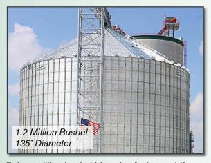
Sukup million bushel bins also feature a 14' or 20' flat deck around the peak of the bin. This provides more area to attach catwalks and conveyors as well as more room to work, making it safer to service.
