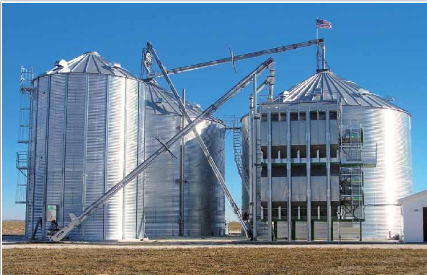
Stationary grain Pump filling a dryer and unloading dryer to multiple bins
