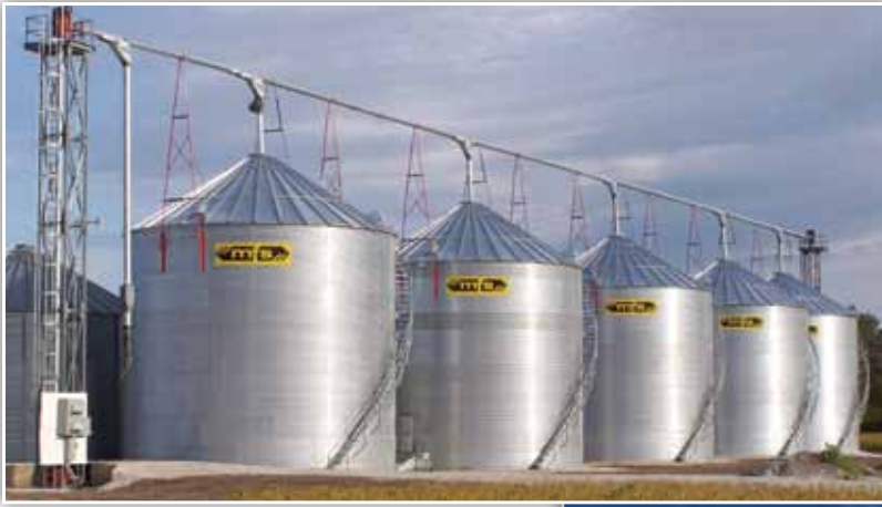
Installation of Grain Pump loop system into a new 5 bin structure.
