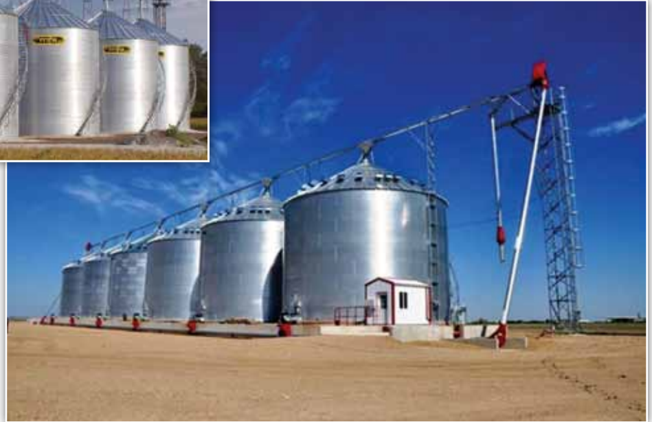
Installation of Grain Pump loop system into existing bin structure
